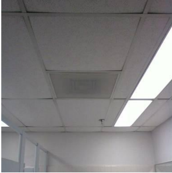
Figure 64 – Ceiling tile representative of 1990's interior finishing, including fluorescent lighting.
