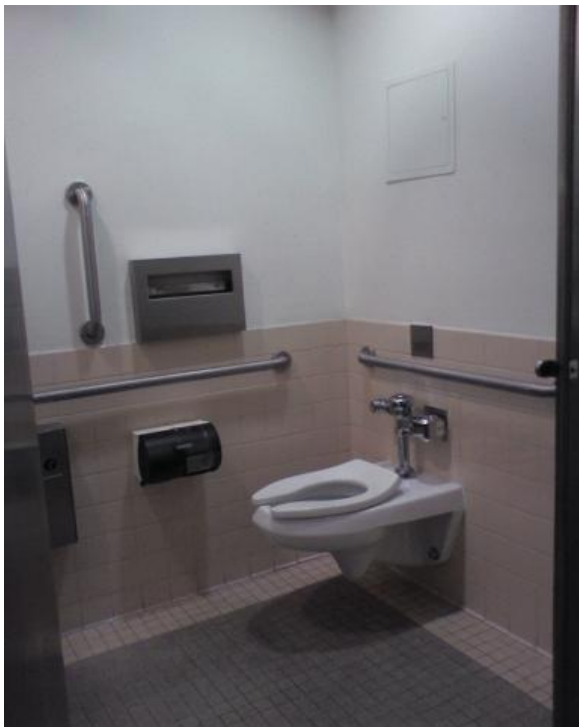
Figure 68 – ADA Wheelchair accessible water closet at 1 st . Floor women's restroom.
