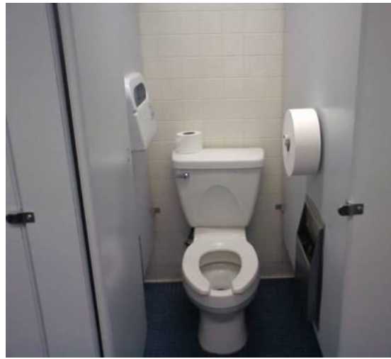
Figure 63 – Dated plumbing fixtures is the case at Women’s Second floor restroom.
