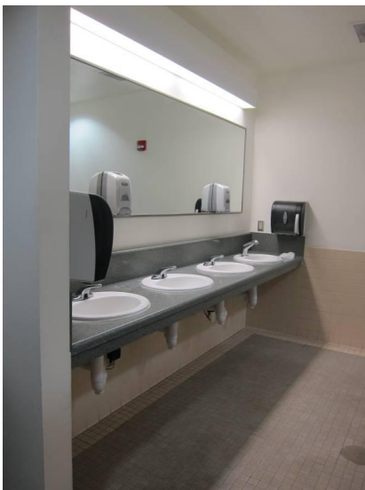
Figure 58 – 1 st . Floor Men's restroom recently remodeled.
