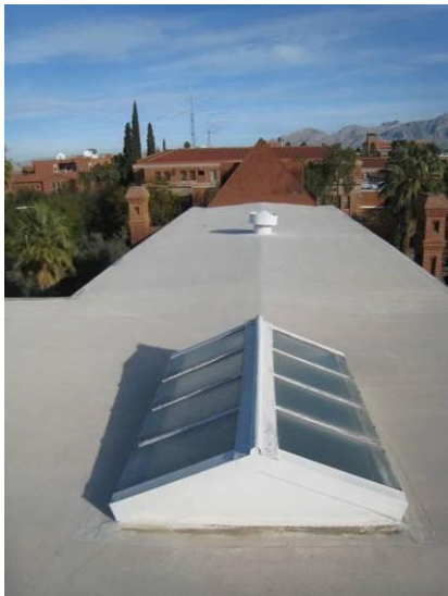
Figure 7 - North skylight at center of hallway.
