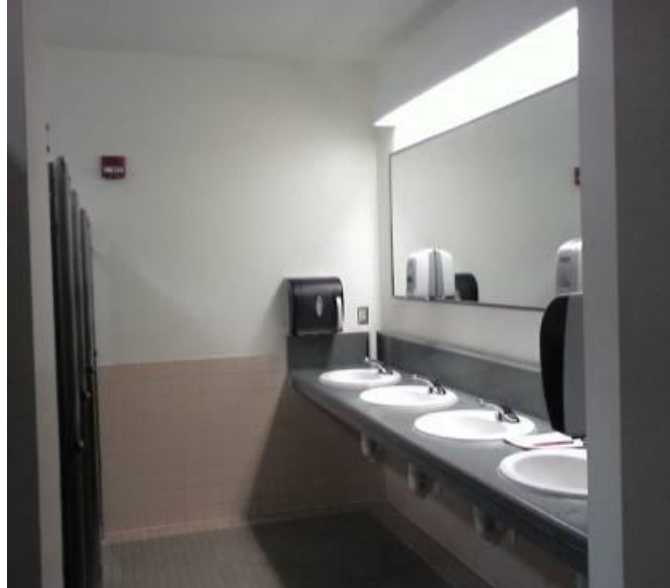
Figure 61 – 1 st . Floor Women’s restroom, showing washbasin counter, with motion sensor faucets and newer materials.
