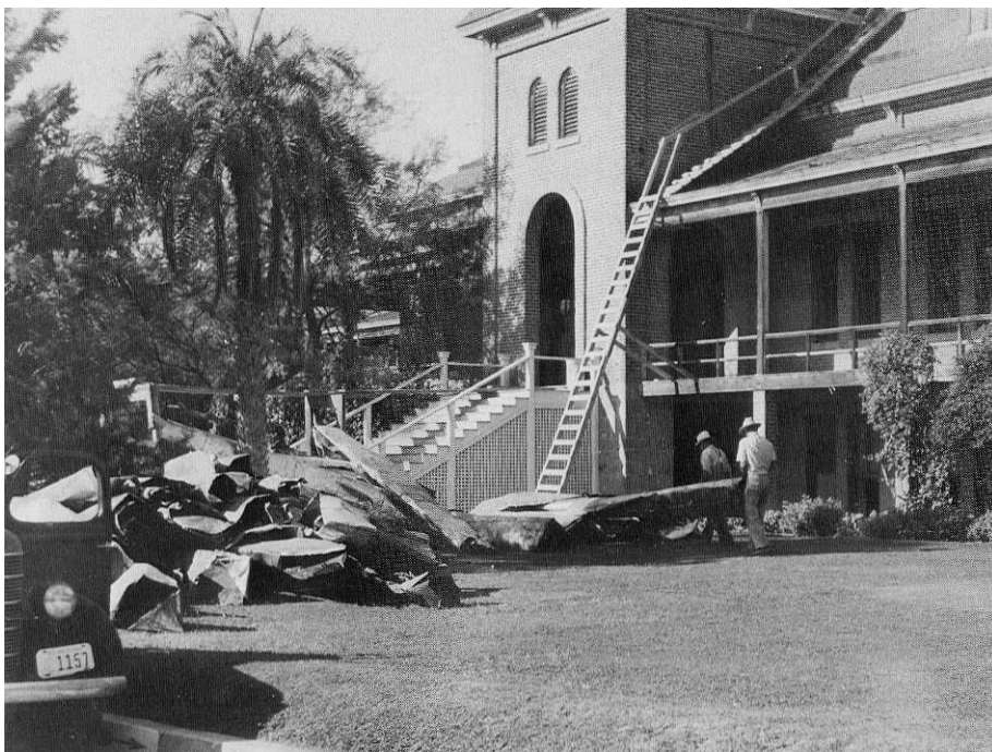
Figure L - Standing seam metal from central roof removed in September 1942 by Sundt Construction Co. in renovations carried out for the Navy at the start of WW2.
