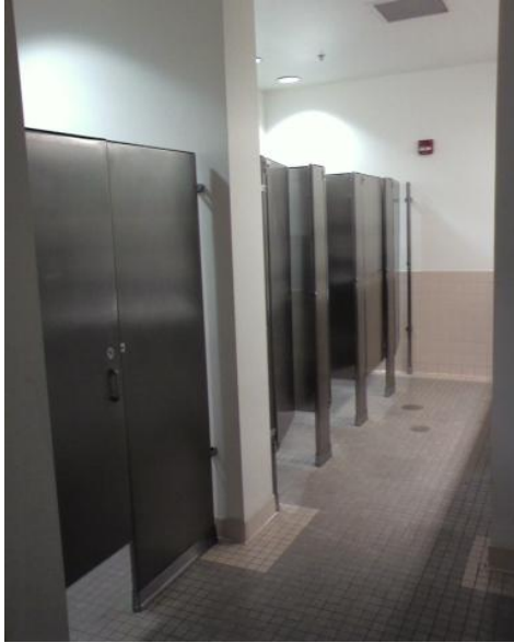
Figure 60 – 1 st . Floor Women’s restroom, showing four individual water closets at far end, and one ADA accessible water closet separated by partition wall.
