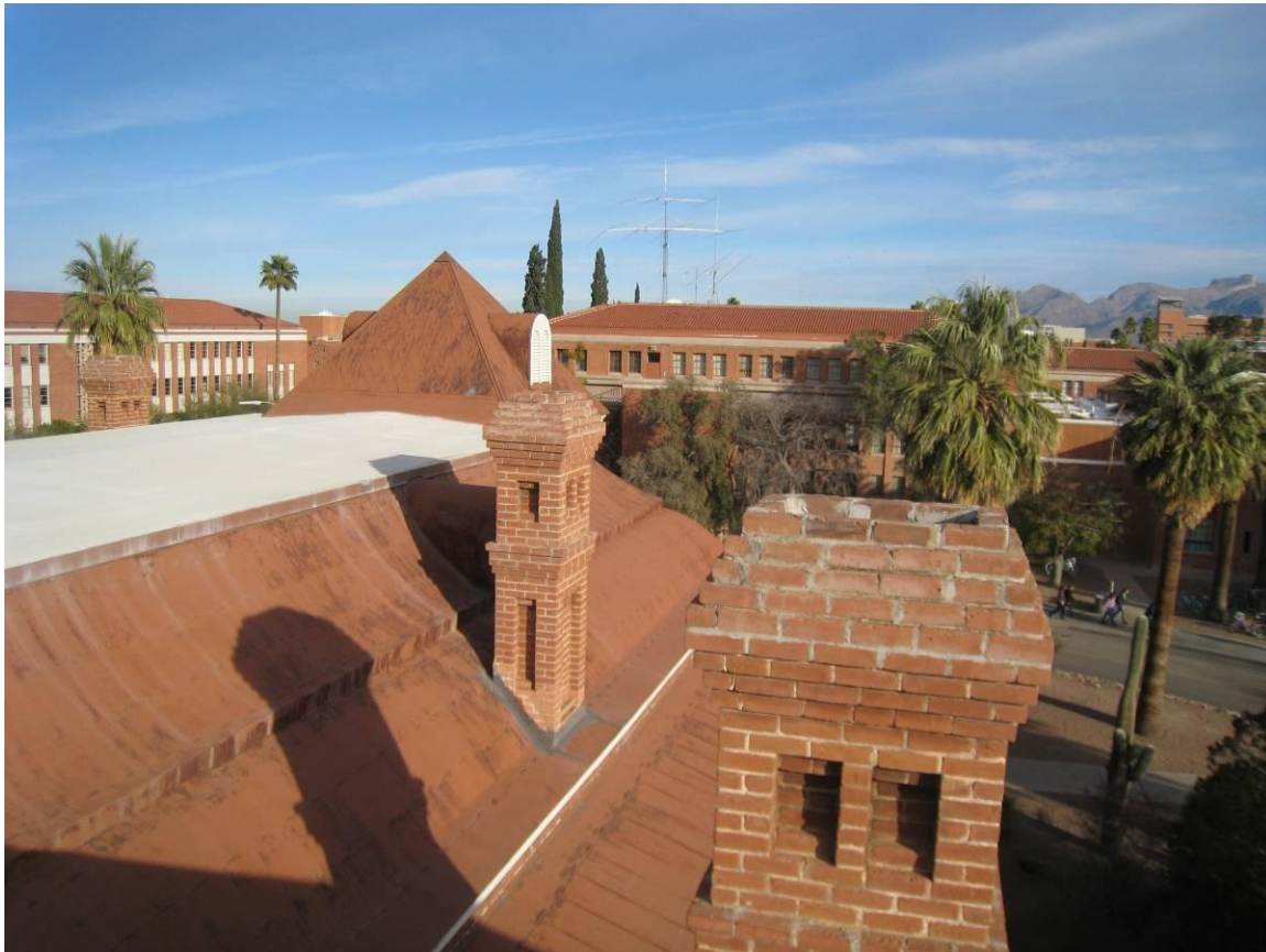
Figure 2 - East side of roof looking north.(B. Vint, 1/25/11)
