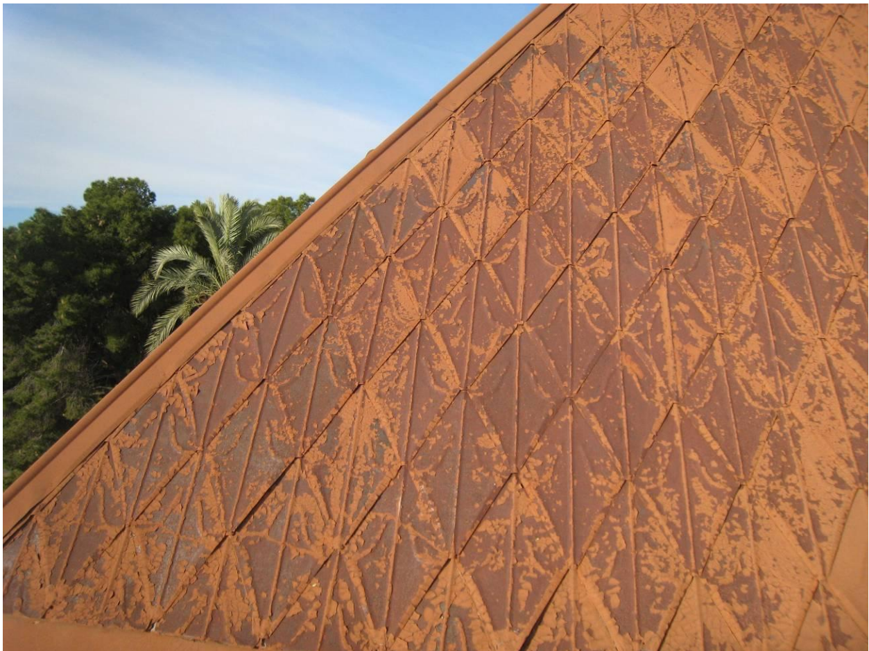
Figure 14 - Detail of terne-metal 'fish scale' roof tiles at West tower.
