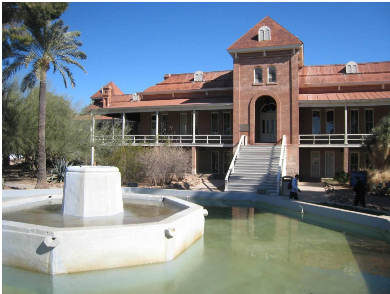
Figure 1- West façade of Old Main with Memorial Fountain frozen solid, 2/3/11 (B. Vint)
