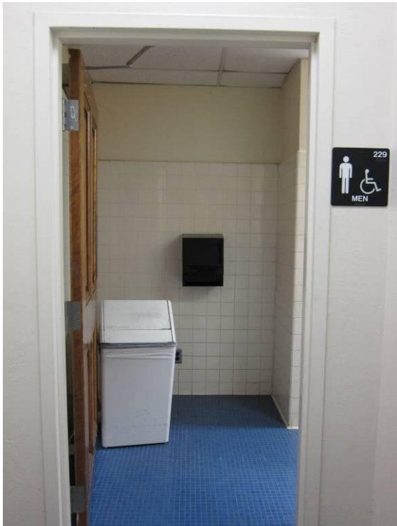
Figure 66 – Second Floor Restroom material palette.
