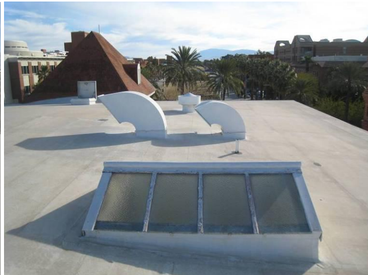
Figure 8 - South skylight with roof hoods beyond, membrane roofing in place.
