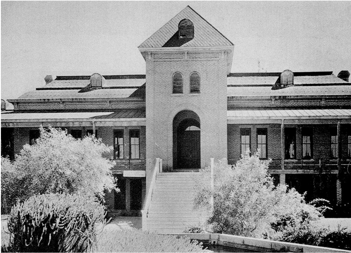
Figure O - West elevation 1938 with Memorial Fountain in foreground overgrown with vegetation. Note weathered and dilapidated appearance of building with pieces missing from wood louvers at ventilation dormers. According to the National Register nomination this was the year that the City of Tucson condemned Old Main as unsafe and University administrators considered demolition. Finials & weathervanes missing from peak of west tower.
