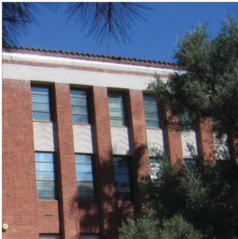
The Harshbarger Mines Building is one of the University's Modern buildings that fits into the Transitional period. The chevron pattern in the spandrels is a character-defining feature of the building.
