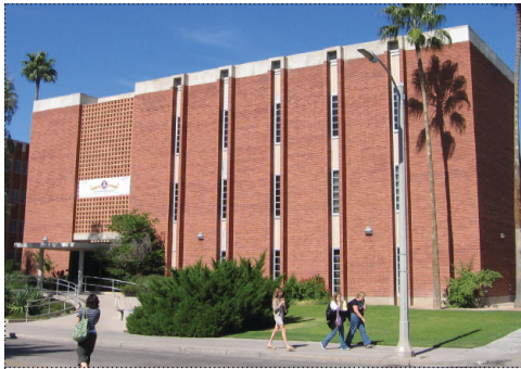
The Civil Engineering Building combines elements of the International Style, such as expression of modern materials and minimal detailing with elements derived from earlier campus architecture, such as tiled spandrels and a simplified base and cornice.
