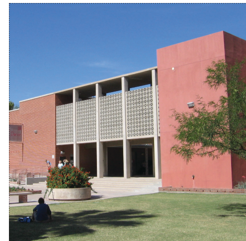
While the Gittings Buildings is unremarkable in its form and materiality, it responds nicely to Tucson’s excellent climate by featuring a large interior courtyard.
