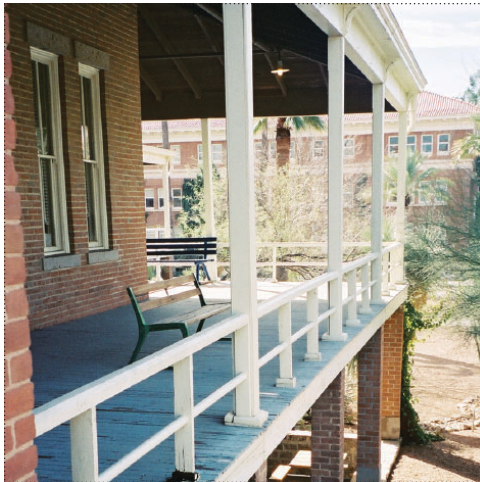
The campus's first major building, Old Main, was one of the last to provide, in the form of a veranda, effective shaded transitional spaces between dark interiors and the unrelenting Arizona sun. While the more Classically inspired later structures sometimes featured a small entry portico, these features were not as effective shade devices.
