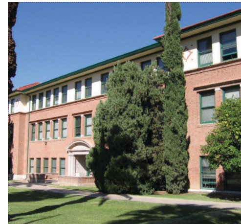
With the construction of the Science Building (now English as a Second Language) in 1909, the City Beautiful movement found its way onto the University campus. The placement of the building to the northwest of Old Main and directly on axis with the 1904 Library gave the campus a more formal arrangement.
