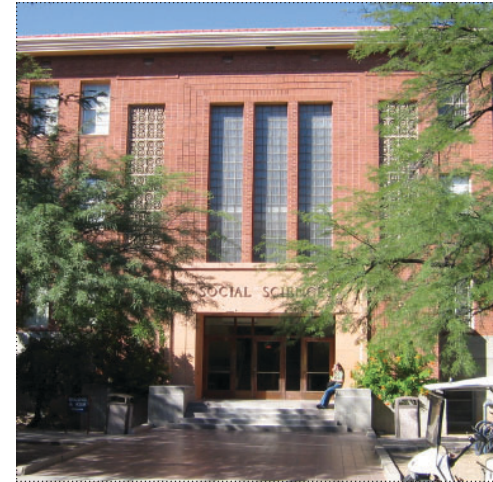
The use of glass block, decorative brick work and concrete block grilles are common elements of the Transitional period. The composition of the central entry at Social Sciences is a clearly Modern expression.
