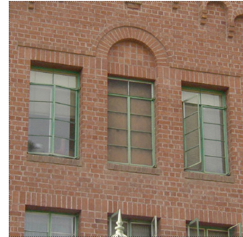
A classic example of steel sash casement windows on the University’s older buildings.
