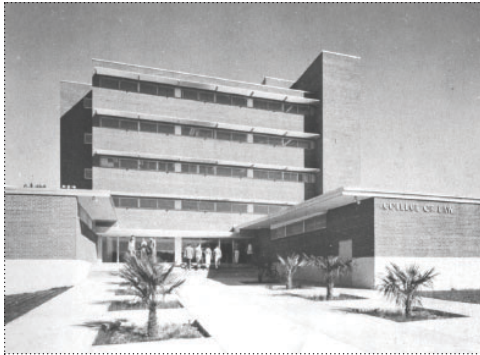
Arthur Brown's Law Building (later Franklin) was demolished in 2006 but it was an excellent example of the asymmetrical massing, ribbon windows, and minimal detailing of the International Style.
